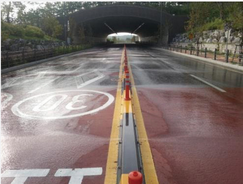
Figure 27 An automatic road-spraying and anti-icing system using rainwater (Source: Suwon City Government, 2013)
