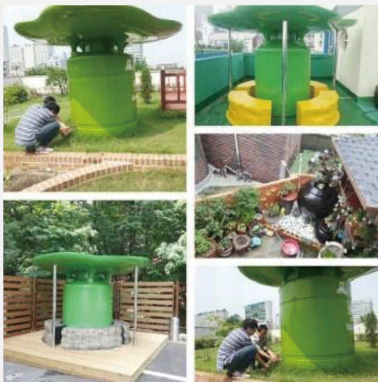
Figure 26 The rainwater collector (Source: (T. Kang, 2014))
